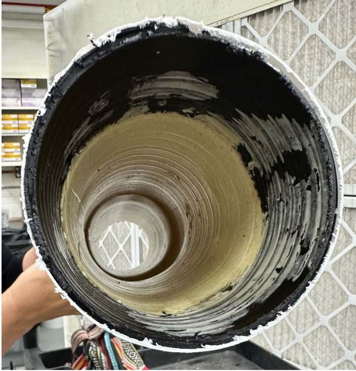
Figure 6. Interior of pipe showing pipe packer structural FRP repair.
